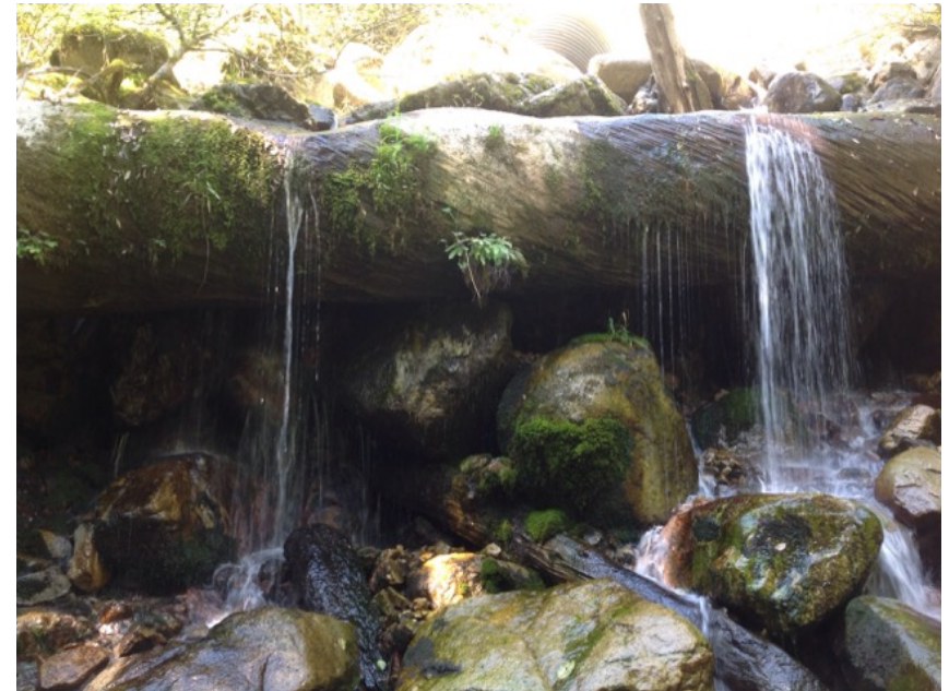
middle of log retaining fill bearing on creek material
