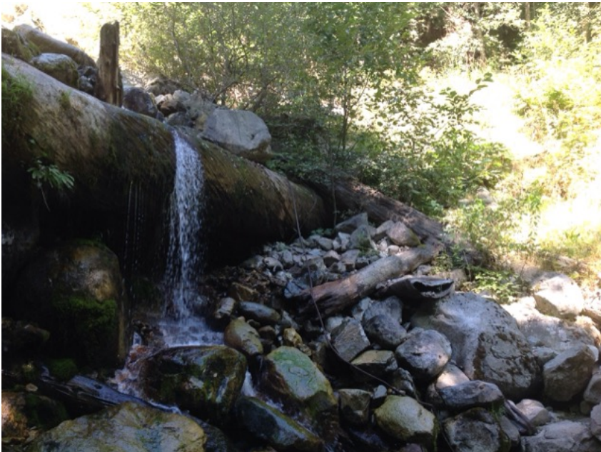
left bank of large log retaining fill appears appropriately tied to bank
