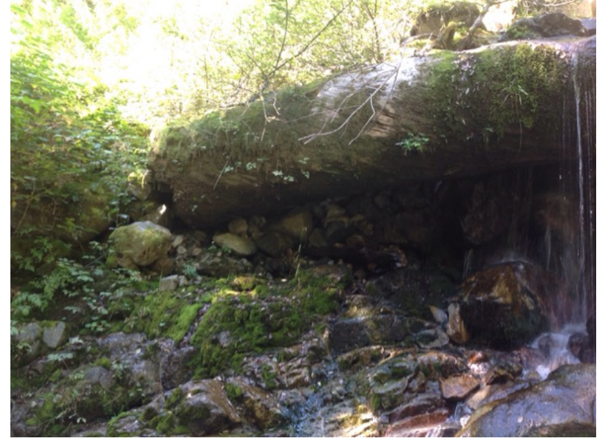
right bank of log retaining fill just sitting on erodible material
