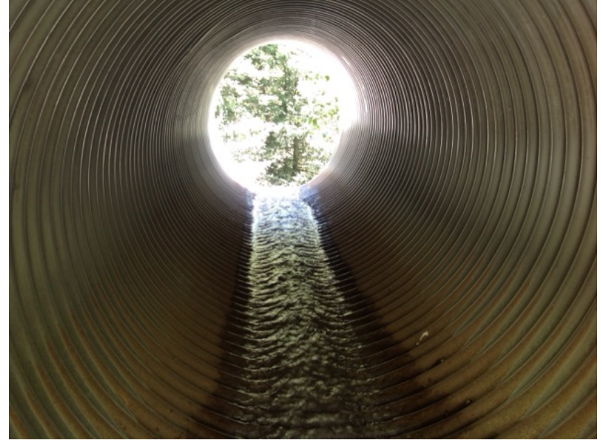
looking through culvert
