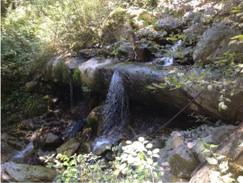
large log retaining fill at outlet
