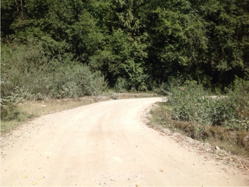
Approach from Right Bank when facing downstream
